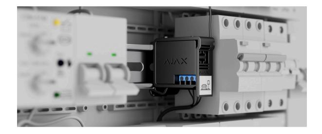
The device is connected to the  $110/230 \text{ V} \sim \text{grid}$ . The WallSwitch dimensions (39 × 33 × 18 mm) allow installing the device into the deep junction box, inside the electrical appliance enclosure, or in the distribution board. A flexible external antenna ensures stable communication. To install WallSwitch on a DIN rail, we recommend using a **DIN Holder**.
